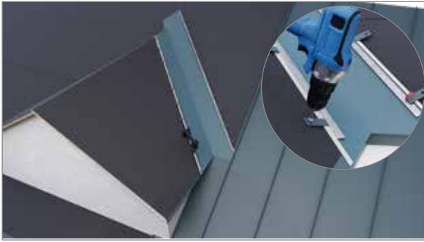
Fold joint around the ridge of approx. 25 mm. Fold the fastening sill over the edge and fasten with screws. These will be the valley channel's fixing points in the roof.
