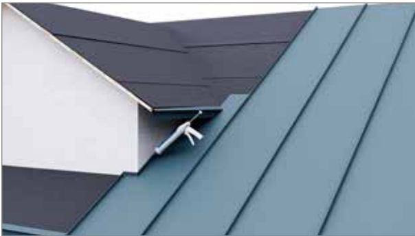
Apply a bead of sealant at the fold towards the ridge.
