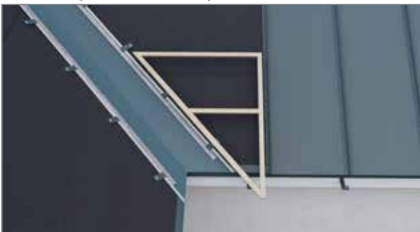
Measure the angle by making a template from wooden studs.
