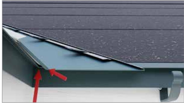
Position the valley channel in the valley so that its fold hooks onto the FSRP eaves board.
