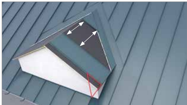
Cover with a temporary roof sheet to the left of the valley and make sure that it is aligned with the eaves board. Use it to measure. Then cover from the valley. Remove the temporary roofing sheet.
