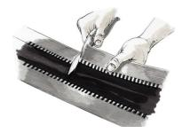
At a notch, cut a length equivalent to the perimeter required plus an overlap of 5 to 6 cm for joining
